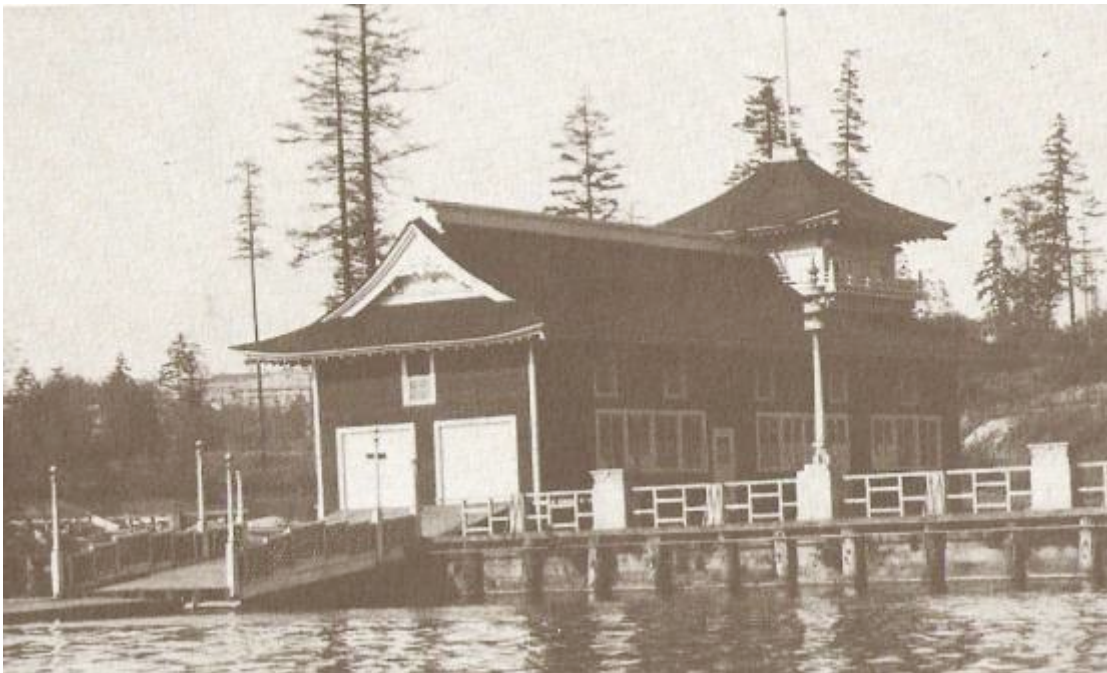
(Tokyo Tea House used as boat building shop by George and Richard Pocock)
